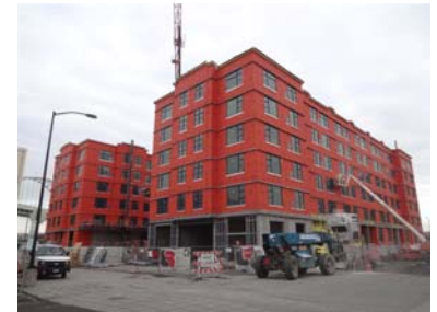
Under Construction 177 Unit The Parker Apartments 1415 NW 12th Avenue
