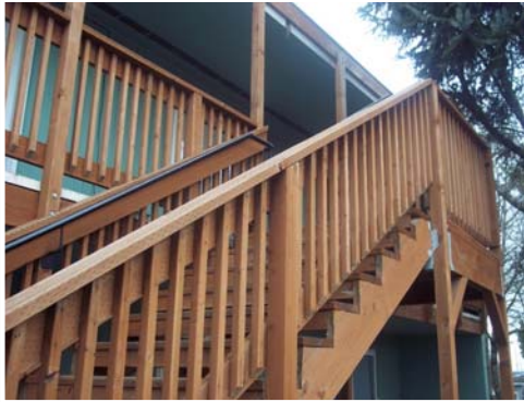
New Long-boarded Railings
