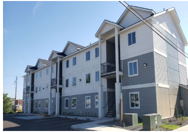
Fiske Apartment Building 1606 N Fiske St Spokane, WA 99207
