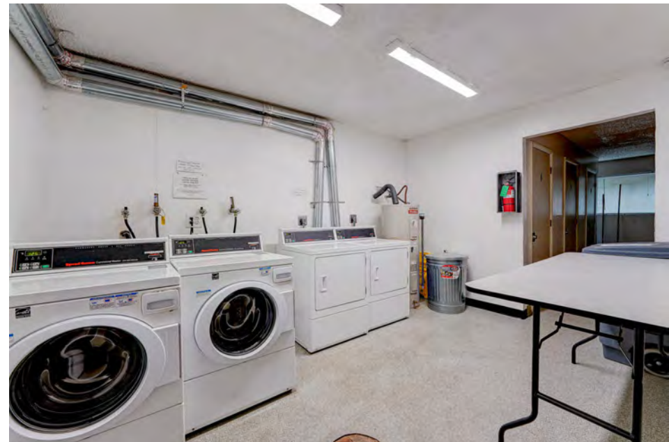
Laundry Room 2, with additional storage lockers
